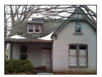
What was once a great example of Gothic Revival architecture has become a worsening eyesore. The house, which features a high pitched gable roof and ornamental brackets, is slowly succumbing to structural failures in the roof, walls, porch, and rear addition. Its condition is severe enough that it could be considered a "demolition by neglect". (On Endangered Buildings List since 2015)
